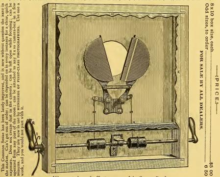
[Above cut shows the Shutter INSIDE of the Camera Box.]
